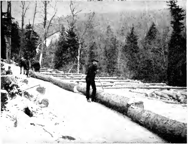
FIG. 33. — A Turn of Logs at the Dump along a Skipper Road. The logs are fastened together with "single coupler" grabs. West Virginia.
